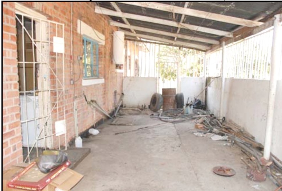
The house entrance through a secure patio
