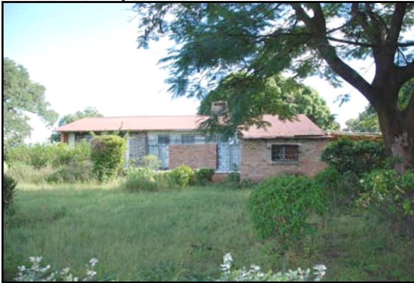
The house at Stand 105 Thorite Avenue, Itimpi, Kitwe
